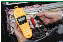
Telephone line testing
